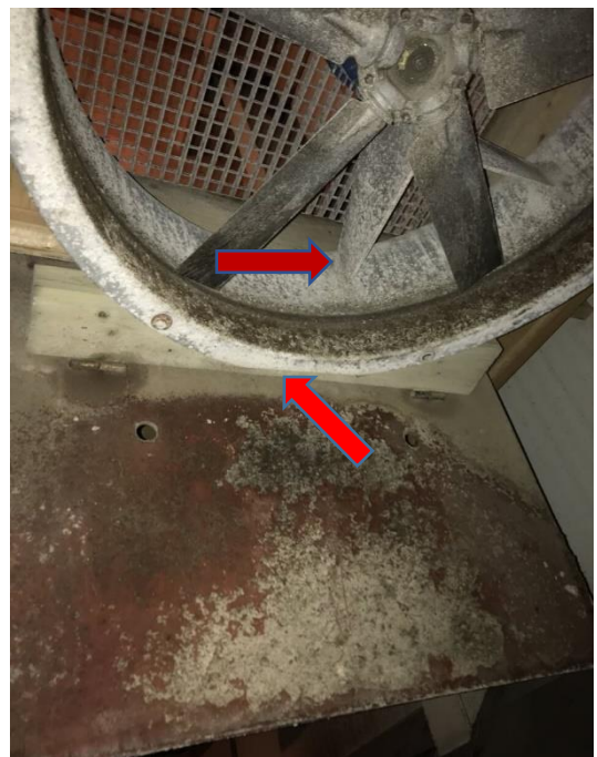
Figure 3 - Fan and its wooden reverse airflow cover with CIPC deposits
