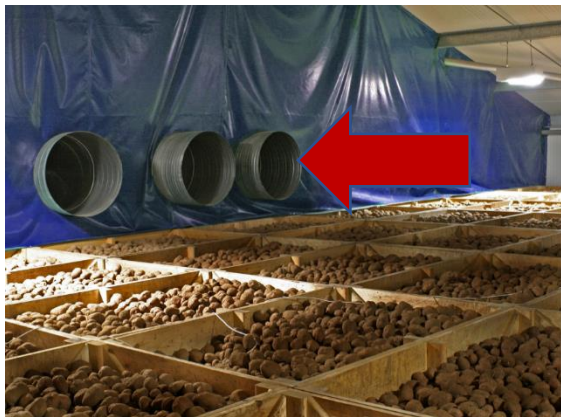
Figure 5&6 Air cooling equipment and associated ducts in box stores
