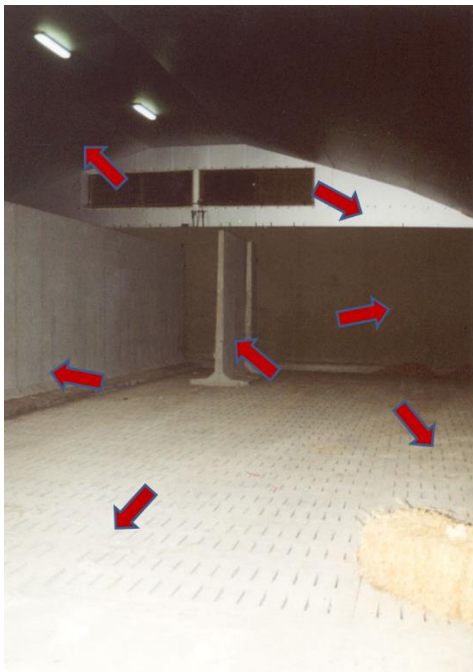
Figure 2 - Places of the store where CIPC contamination can be easily demonstrated
